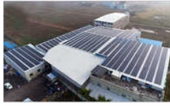
300 KW Trunkey Project
