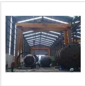
Traveling Goliath Crane
