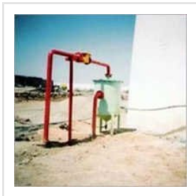
Biogas Treatment Moisture Traps
