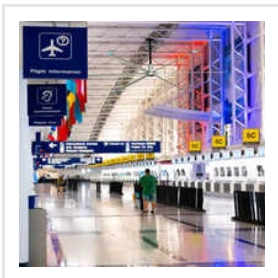
Airport HVLS Fans
