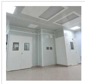
Hospital Clean Room
