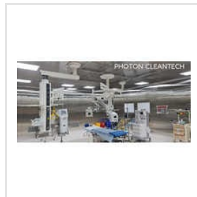
Hospital Modular OT
