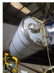
Stainless Steel Tank Installation Services
