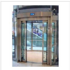
Shopping Mall Elevator
