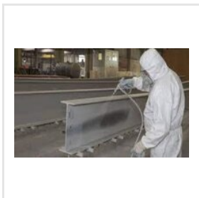
Anti Corrosion Coating
