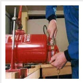
Hydrant System Maintenance Service
