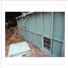
Fabricated Platform Tata Steel Furnace
